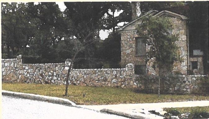
Stone walls of varying heights and designs are found in many of San Antonio's historic districts. In some locations (as illustrated above), the walls are used to enclose and screen a yard. In other locations, lower stone walls are used for retention purposes on sloped sites.
